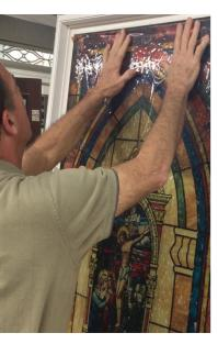
7. Carefully place your film on your glass and slide it into place making sure you hand smooth out any large bubbles from the back the soapy spray should allow you to freely glide the film over your window.
