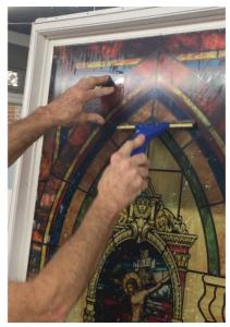
8. Squeegee a small section of film, up top. Start with minimal pressure, then add more pressure as more air and bubbles are pushed out. Spraying the front of your film makes this step easier allowing the squeegee to glide over the film easily
