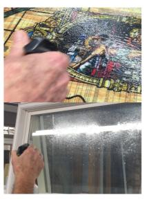
6. Carefully transport your film sticky sprayed side away from you to your wet window. Walk carefully enough to keep the film steady, (which makes the next step easier)
